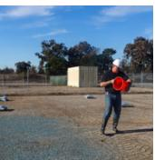
For erosion control contractors, installation of traditional hydraulically spray applied erosion control products is challenging due to tight spacing limiting hydroseeder access and overspray soiling the panels. EDGE™ EarthGuard® Pellets are a solution that can be applied easily between solar panel rows.
